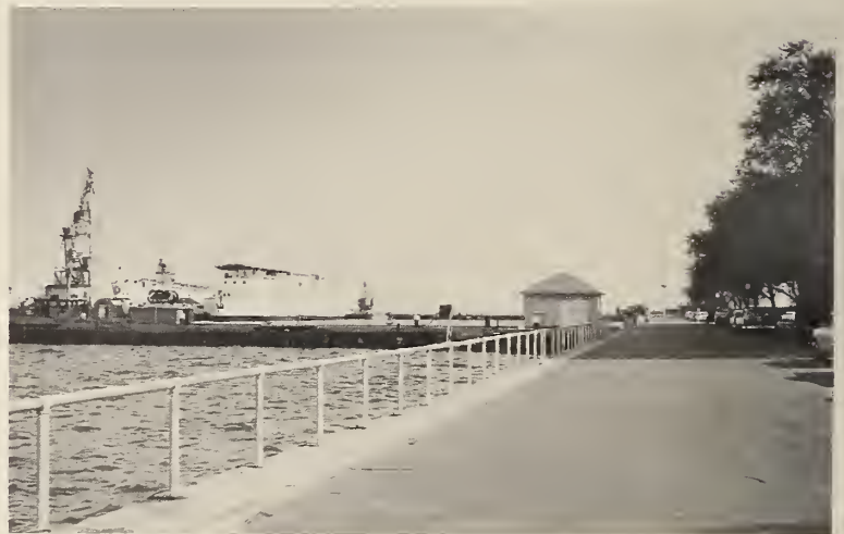
Along the seawall.
